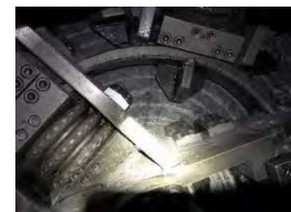
(4工区)地山岩盤確認
